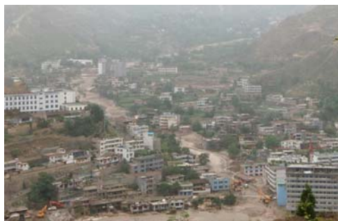
Debris flows at Sanyanyu and Luojiayu Gully ruined the city
