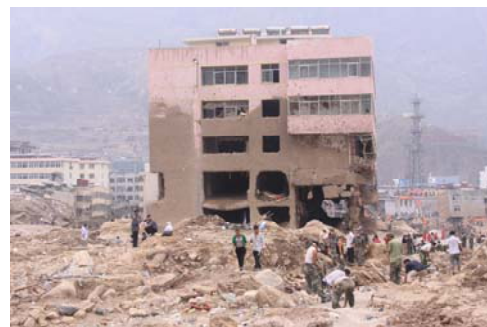
The building was damaged
